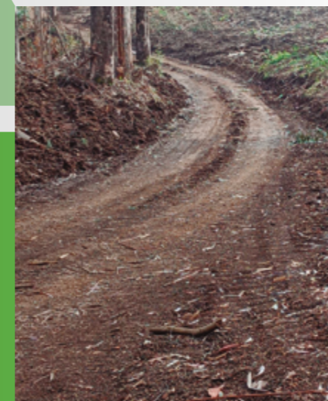
Road maintenance — Sincol
