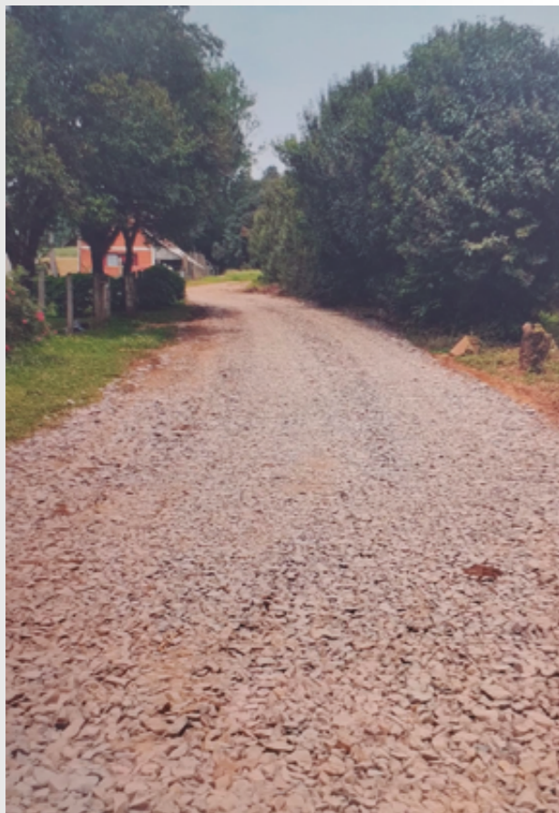
Road improvements on the Horizonte I farm
