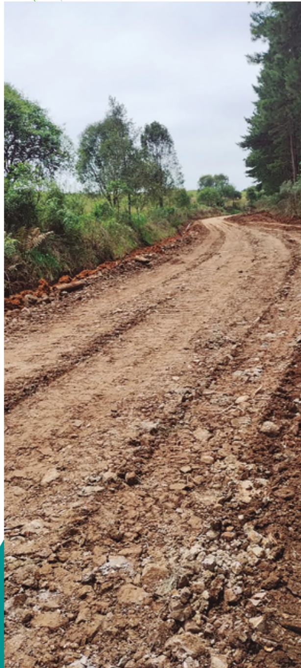
Road improvements on the Sincol farm
