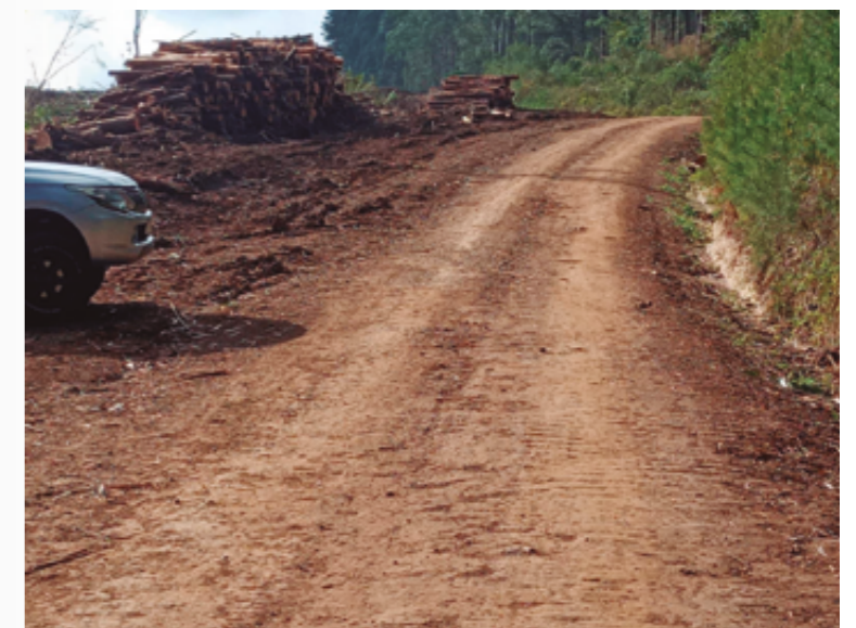
Road maintenance — Horizonte I
